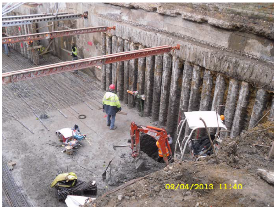
Figure 18. Contiguous bored pile wall
