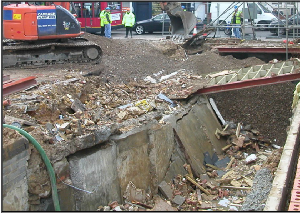
Figure 7. Effect of horizontal force from the ground on unrestrained basement wall
