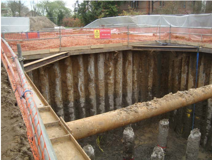
Figure 33. Bottom up construction
