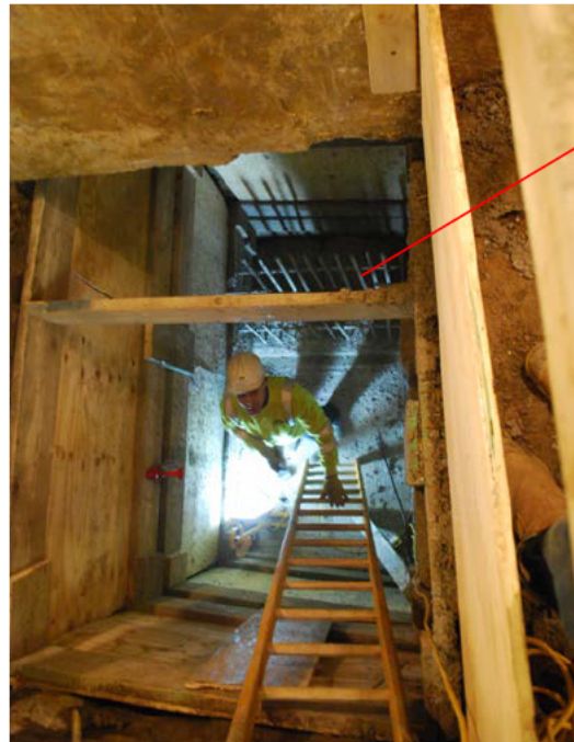
Figure 6. Underpinning
