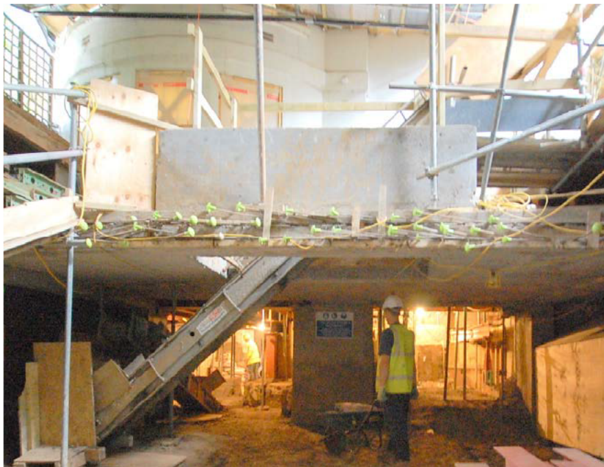
Figure 37. Tunnelling under occupied house
