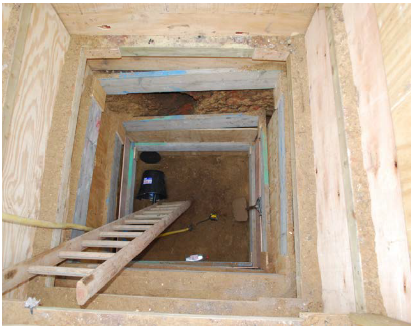
Figure 28. Temporary works - individual underpin
