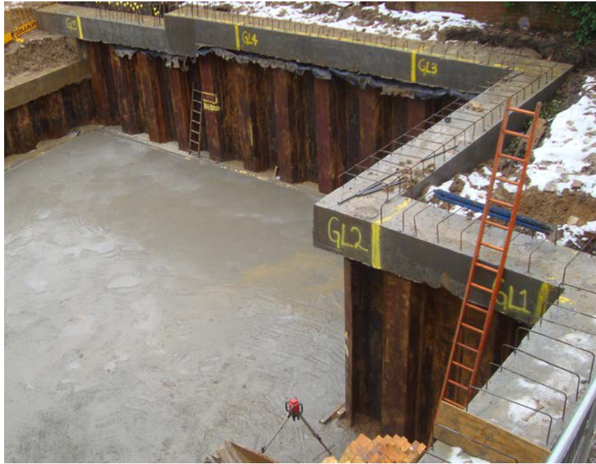
Figure 23. Steel sheet piled wall
