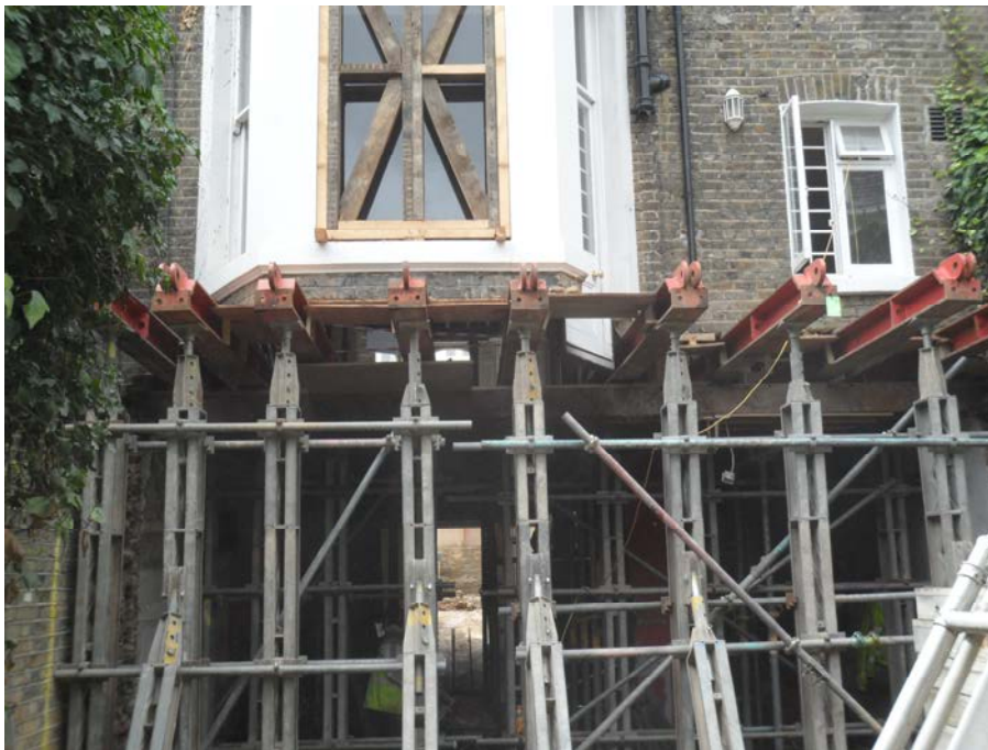
Figure 31. Temporary works - support to existing structure
