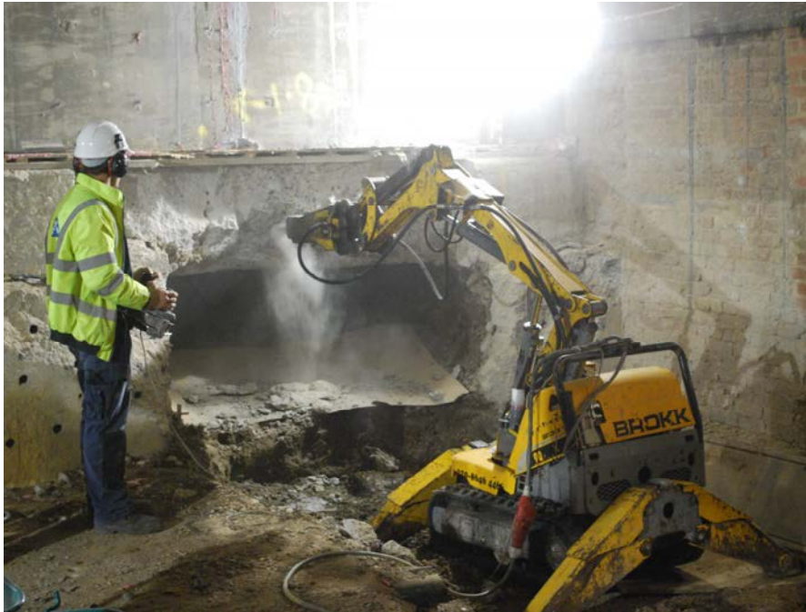
Figure 42. Concrete break out
