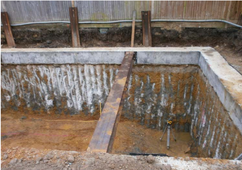
Figure 20. Secant piled wall
