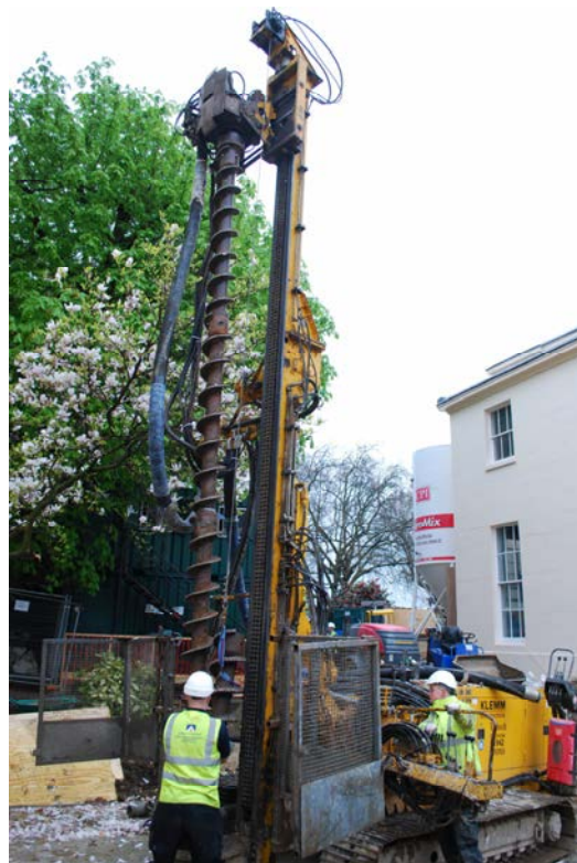
Figure 15. Piling rig in rear garden
