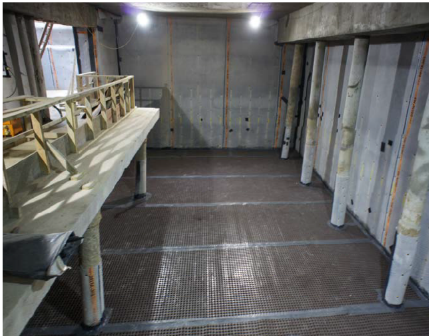
Figure 47. Cavity membrane after installation in a basement
